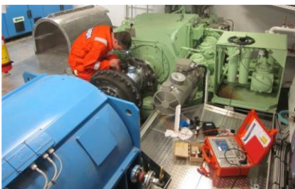
Installation of measuring equipment in engine room
